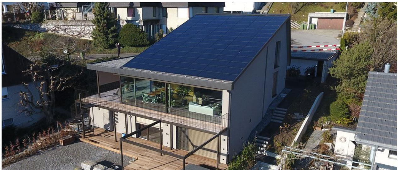
PVA 3S Swiss Solar Solutions – MegaSlate – 18kWp – Indach – Steffisburg - 2019
