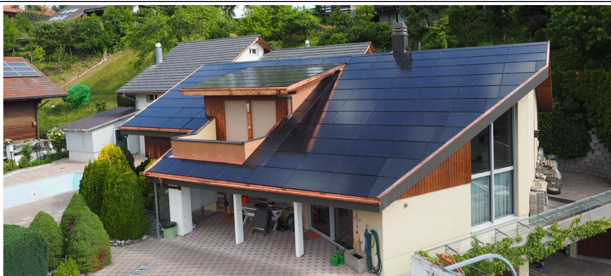
PVA 3S Swiss Solar Solutions – MegaSlate – 24kWp – Indach – Thierachern- 2022
