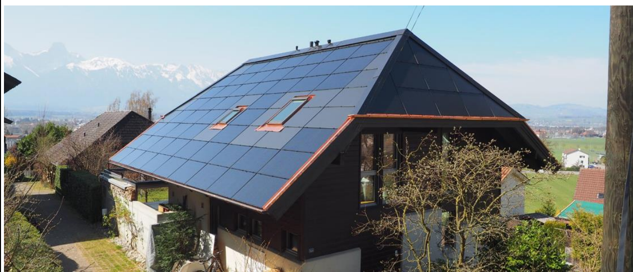
PVA 3S Swiss Solar Solutions – MegaSlate – 22kWp – Indach – Steffisburg - 2020
