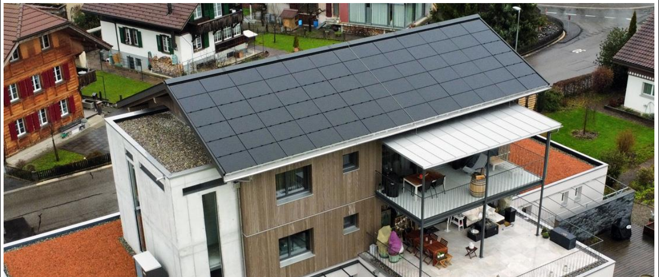
PVA 3S Swiss Solar Solutions – TeraSlate – 17.1kWp - Indach - Schützenstrasse – Heimberg - 2025
