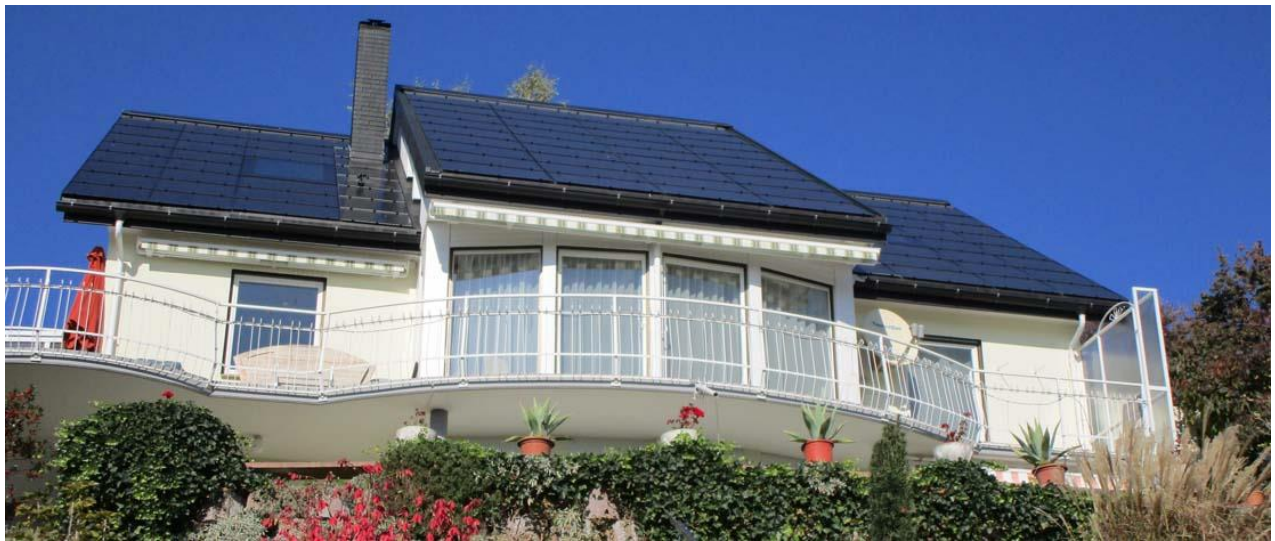
PVA 3S Swiss Solar Solutions – MegaSlate – 13.98kWp – Indach – Steffisburg- 2018
