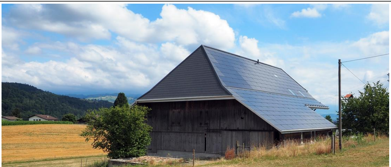
PVA 3S Swiss Solar Solutions – MegaSlate – 100kWp – Indach – Heimberg - 2014
