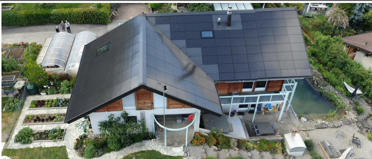
PVA 3S Swiss Solar Solutions – MegaSlate – 27.60kWp – Indach – Hondrich - 2019
