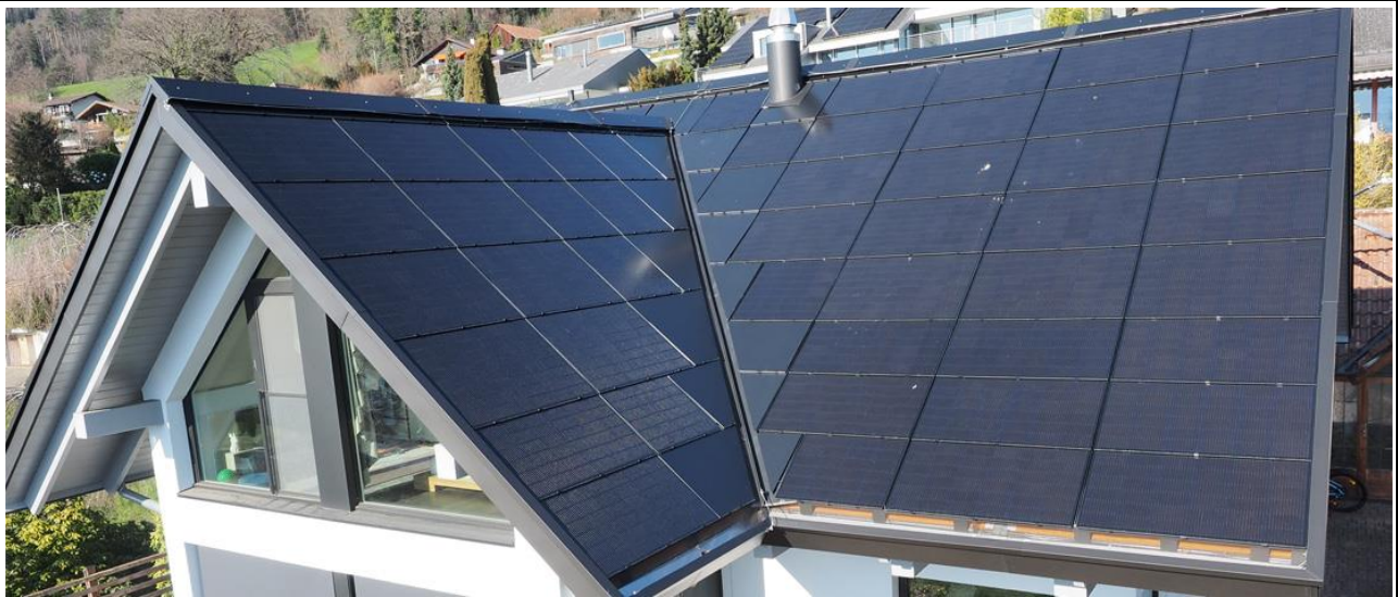
PVA 3S Swiss Solar Solutions – TeraSlate – 28.55kWp – Indach allseitig – Hilterfingen - 2024
