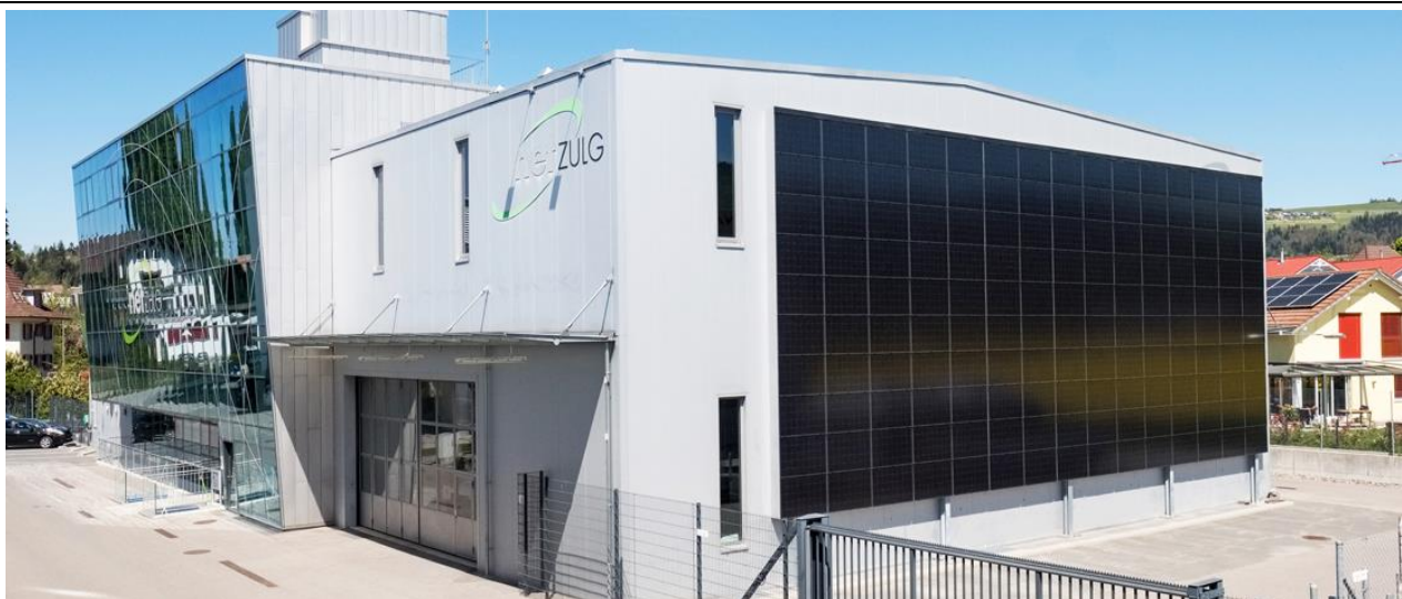
PVA 3S Swiss Solar Solutions – MegaSlate – 28.50kWp – Indach Fassade – Thierachern- 2017
