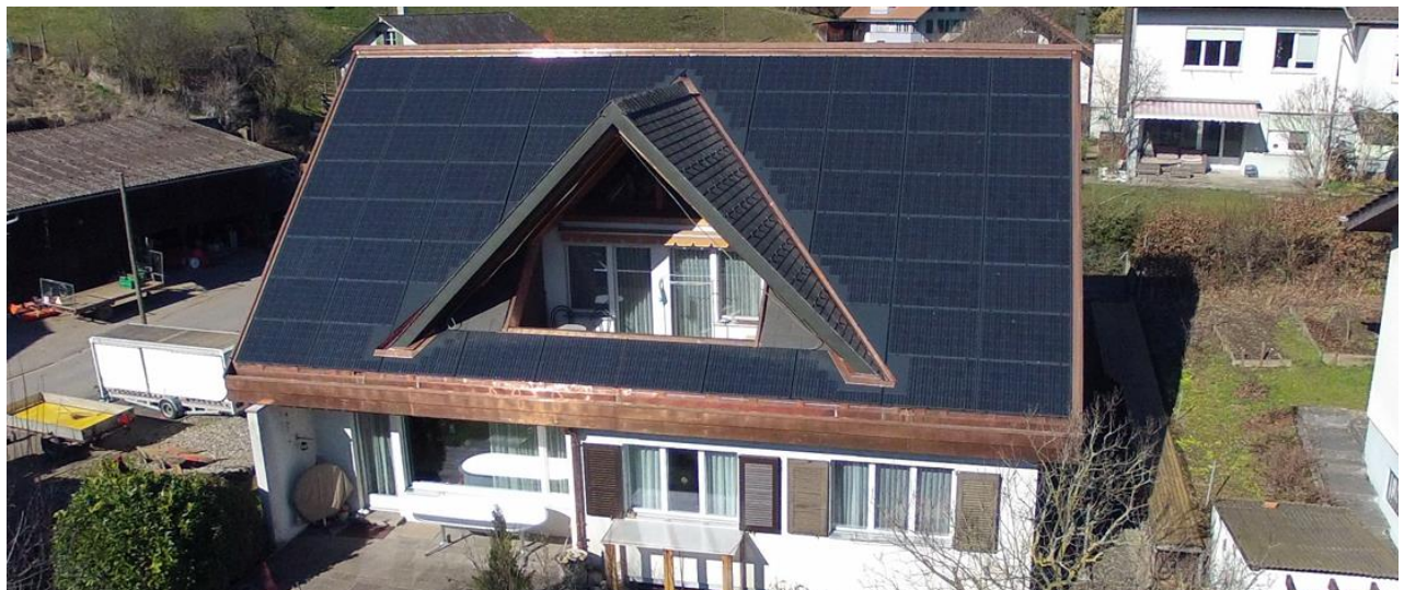
PVA 3S Swiss Solar Solutions – MegaSlate – 9.66kWp – Indach – Uttigen - 2013
