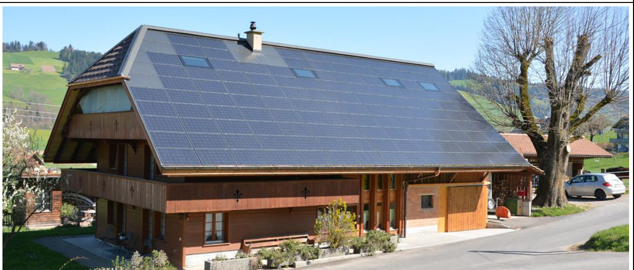
PVA 3S Swiss Solar Solutions – MegaSlate – 23kWp – Indach - Dachfenster – Hinterkappelen- 2015
